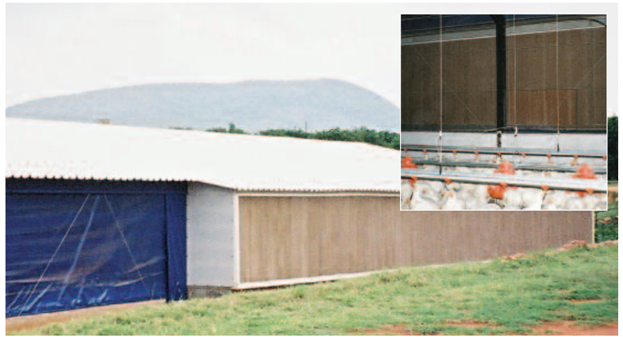
Each building has CELdek® evaporative cooling pads along each side, measuring 1.5 by 16.2 meters.
