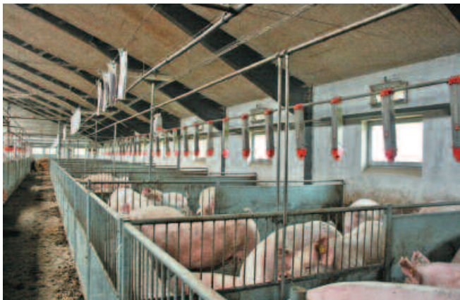
Building A with the IW inlets mounted on the side wall.
