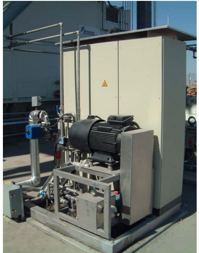
Field installation of Turbofog system for GE LM 6000 gas turbine (1.0 kg/s)
