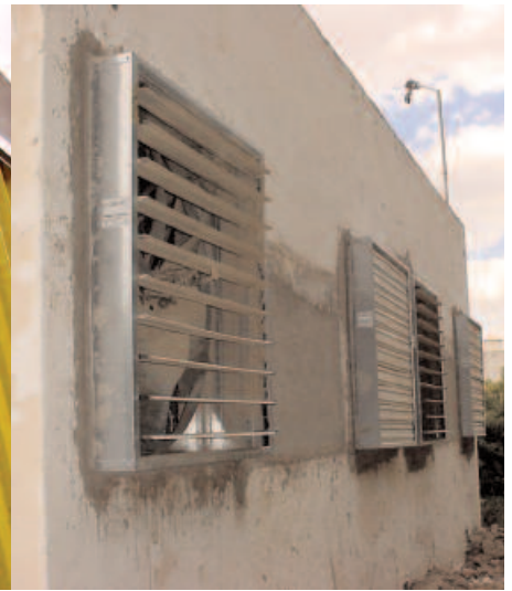
Cooling part of the system (left) with CELdek evaporative cooling pads and ventilation part of the system (right) with Euroemme extraction fans.
