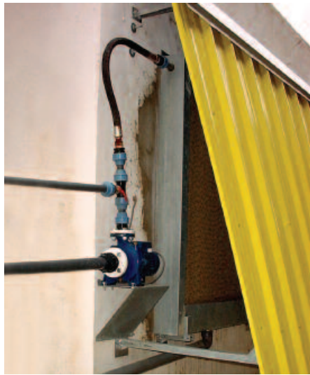
Cooling part of the system (left) with CELdek evaporative cooling pads and ventilation part of the system (right) with Euroemme extraction fans.
